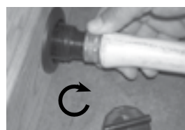
3. Thread hose onto the spa drain
