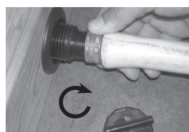
3. Thread hose onto the spa drain
