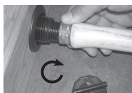
3. Thread hose onto the spa drain
